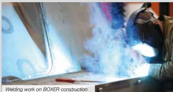
Welding work on BOXER construction
