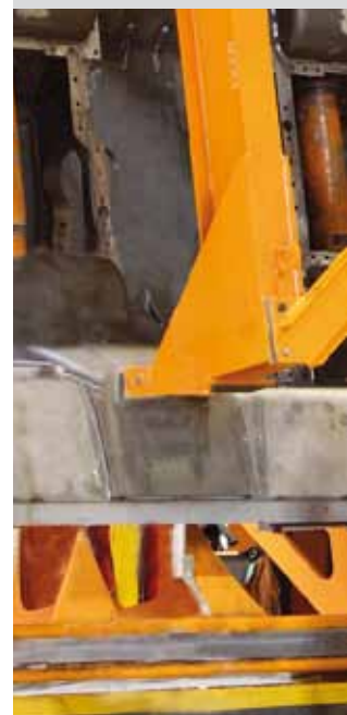
Production facilities for armour plates welding
